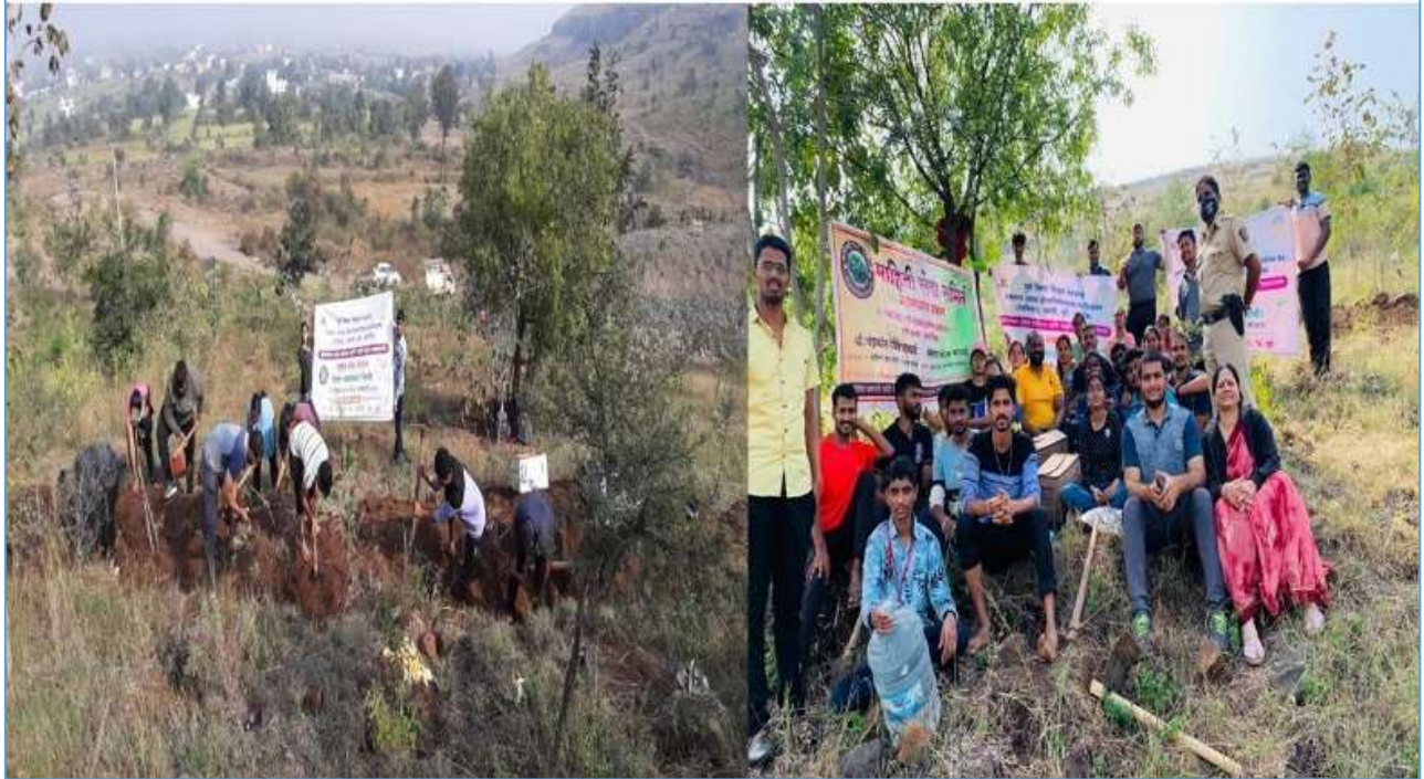
Work for the purpose of water conservation and water horizontally by digging continuous counter trenches(CCT) on the Bakori hills
